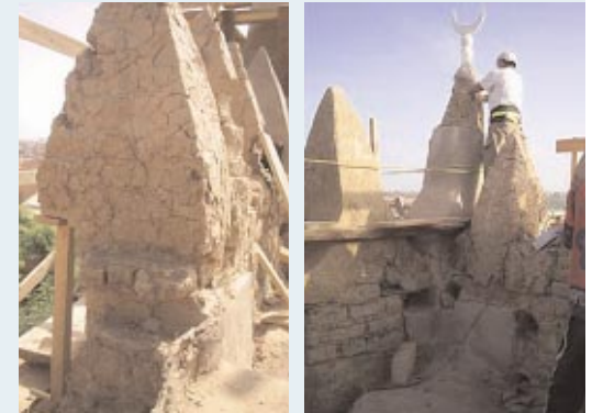
(Left) The exposed parapet pillars following removal of the cement.
